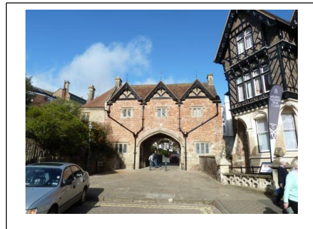
Priory Gateway South side
